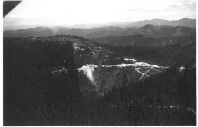
Figure 3. Formosa Resources' Silver Peak Mine (Mine site 23, Table 2) is producing copper, zinc, silver, and gold. Mill and settling pond are located on the ridge crest, and ore is trucked to the mill from the portal at left.
