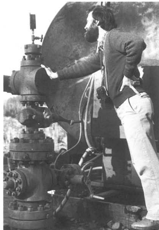
Dennis Olmstead checking pressure gauge at a disposal well in Mist Gas Field.
